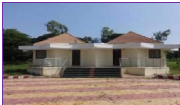
Guest House at Chakur Campus
